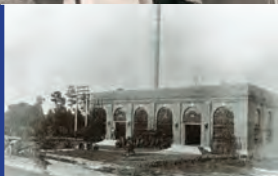
The city-owned downtown power plant was completed.
