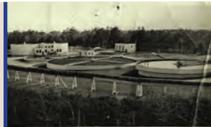
The Main Street Wastewater Treatment Plant offered sanitary sewer service.
