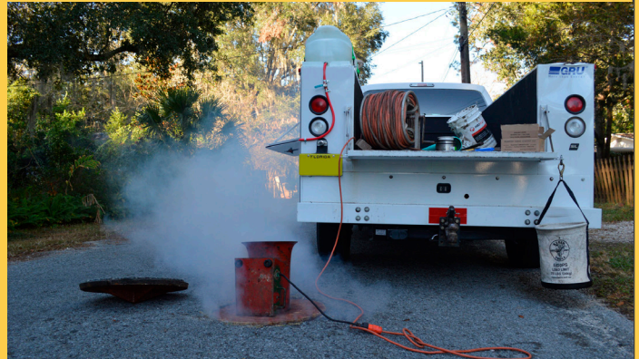
Crew members blow non-toxic smoke into manholes.
