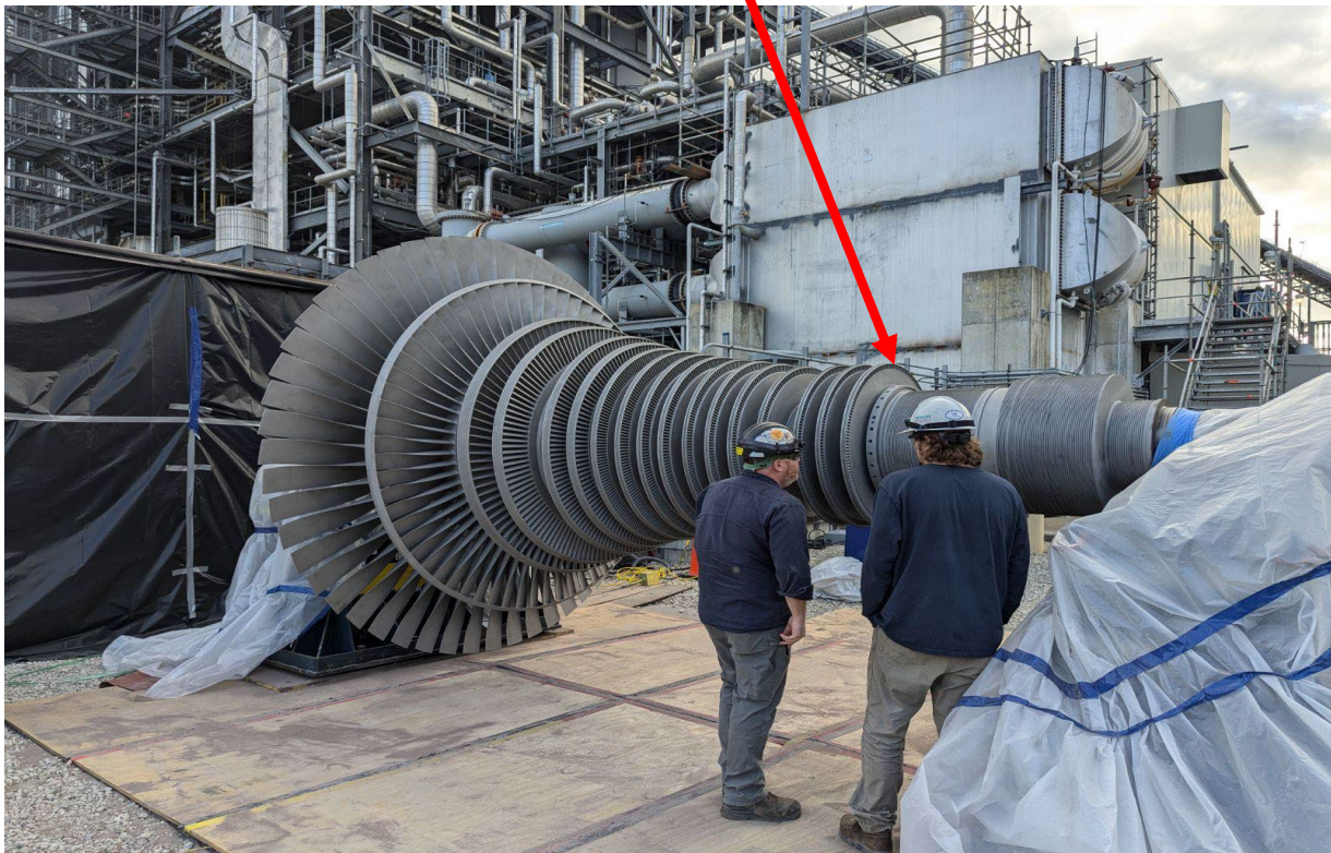
Siemens contractors setting up for NDE testing of rotor blade rings
