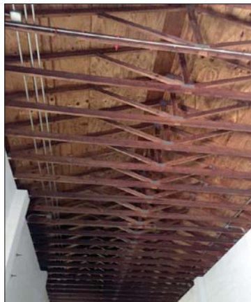
Exposed Roof Structure
