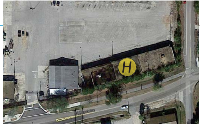
Building H - Water Distribution Construction Building
