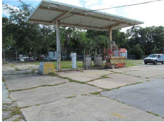
Existing gas canopy
