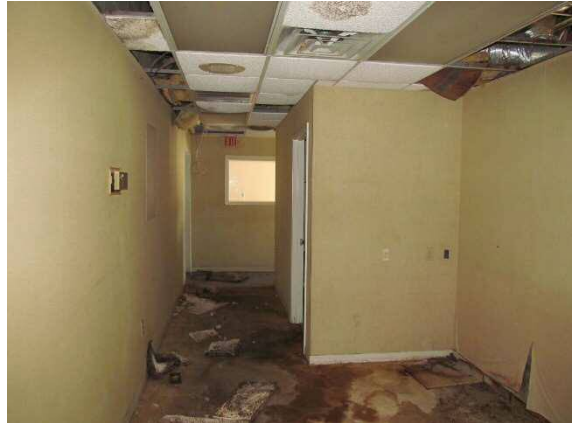
Interior view office area
