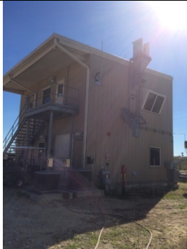
Typical Plant Construction: Fuel sampling and lab building.
