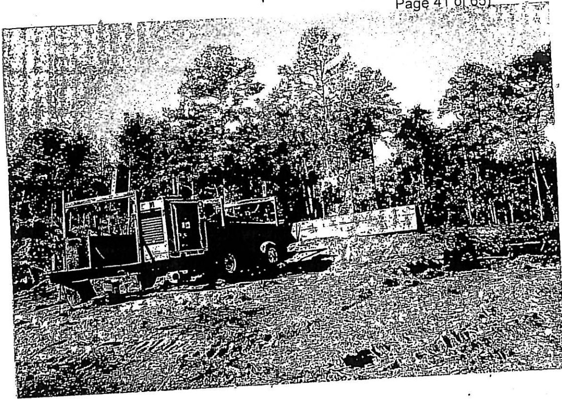
8. 40 FOOT LONG CURTAIN BURNER BEING USED BY WATSON AT THE ST. FRANCIS H.S. SITE
