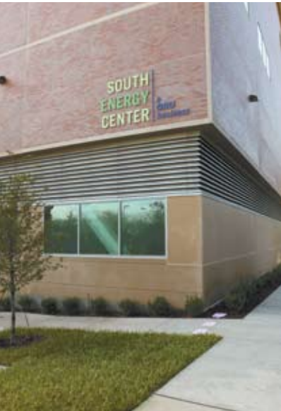
GRU's South Energy Center was dedicated in late 2009.
